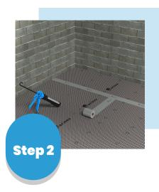
Cover joints with MARMOX Reinforcing Tape. Seal wet areas joints with MS Polymer. Seal with MARMOX sealing tape, if water proofing installation is required.
