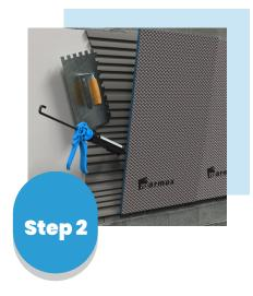
Apply cement tile adhesive all over the surface underneath and the MARMOX BOARD and align the board on the wall. Seal wet areas joints with MS Polymer. If area is dry, then reinforce with fiberglass tape which is embedded in the flexible tile adhesive.
