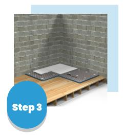
Cover and reinforce joints & holes with fiberglass tape which is embedded in the flexible tile adhesive. Seal with MARMOX sealing tape if waterproofing installation is required. Lay tiles after curing (minimum tile dimension are 100 x 100 mm with thickness not less than 7 mm).
