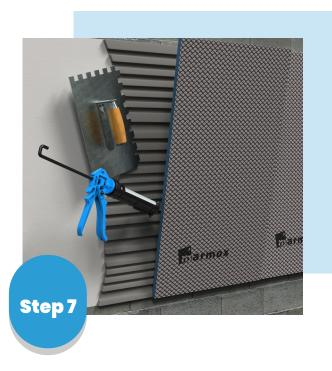
Seal wet areas joints and cover all washers with MS Polymer.
