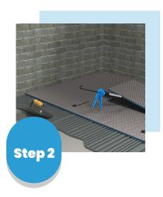
Glue the MARMOX BOARD with flexible tile adhesive in a brick pattern. In wet areas, seal joints with MS Polymer. Apply fiberglass tape which is embedded in the flexible tile adhesive over all joints for reinforcement, with an overlapping of 40-50 mm.
