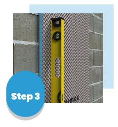
Fix the MARMOX BOARD on the wall at the right position, you may use a rubber hammer to align with the other board. Check that the board is levelled.
