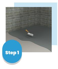
Clean, prime and seal the subsurface before installing of the MARMOX BOARD.
