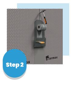
Cover and reinforce joints & holes with fiberglass tape which is embedded in the flexible tile adhesive. Seal with MARMOX sealing tape, if waterproofing installation is required.
