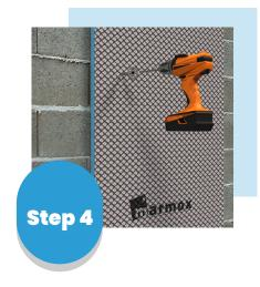
Drill into the substrate through the dabs of adhesive and then position the dowels. Wait for adhesive to cure before hammering the dowels.
