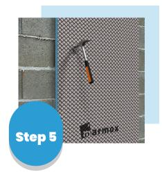
Ensure the penetration of dowels into the load-bearing substructure should not be less than 35 mm.
