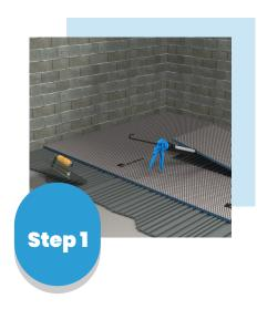
Clean the floor completely. Use a floor trowel to apply a layer of cement-based flexible tile adhesive over the floor. Fix the MARMOX BOARDS down in place and press gently to get them in the right position in a brick pattern.
